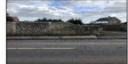
Existing boundary wall along Brannan Road
